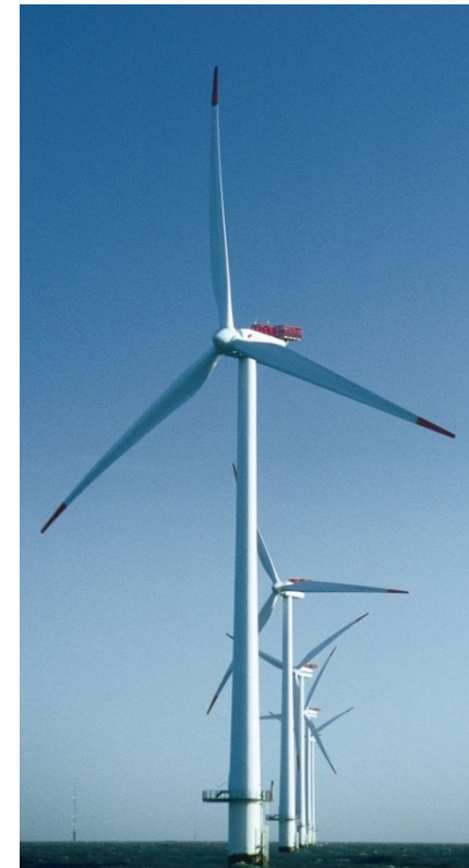
Offshore wind farm
